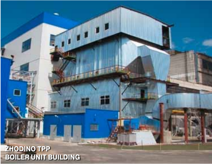
ZHODINO TPP. BOILER UNITBASED ON COMBUSTION OF CRUSHED PEAT AND WOODEN CHIPS MIXTURE HAVING CARACITY 60 T/H FOR STEAM PARAMETERS 9.5 MPA, 5100C.
